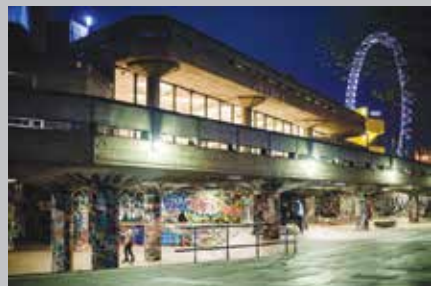
The Undercroft, saved with John's help. Photo: Sam Ashley.
